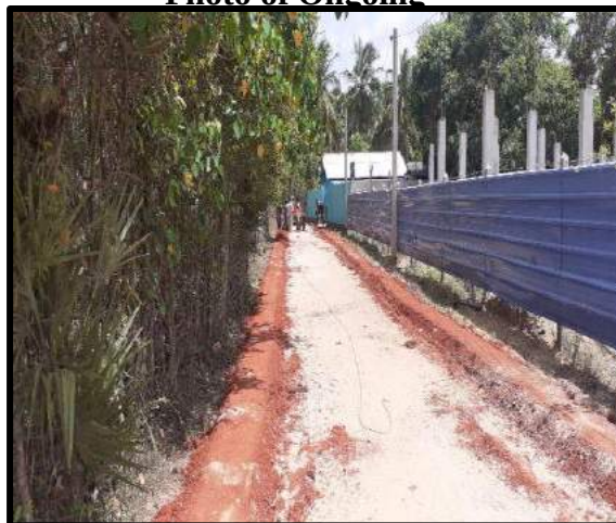
Photo of Ongoing
