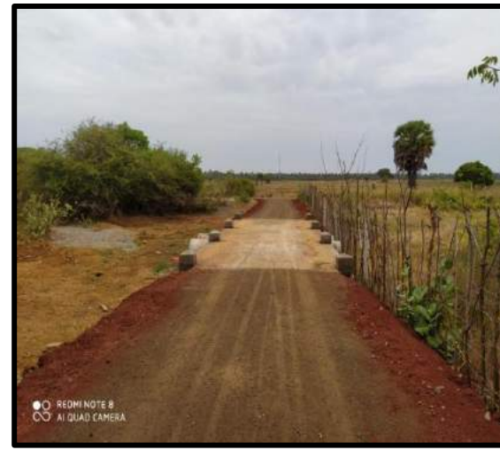
Photo of after the completion
