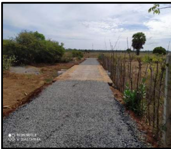
Photo of Ongoing
