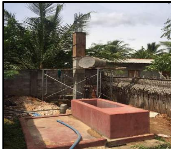
Photo of Ongoing
