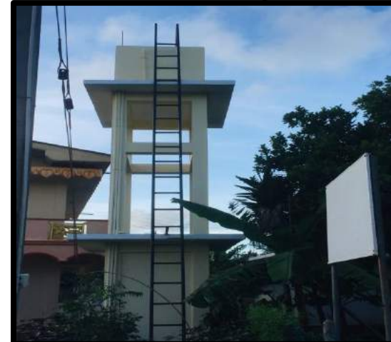
Photo of after the completion
