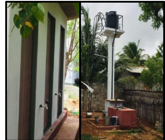
Photo of after the completion
