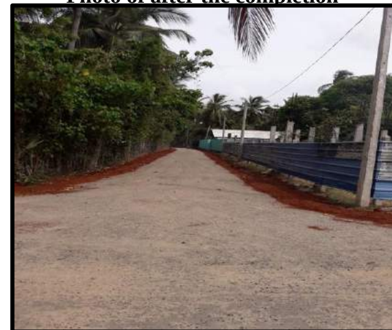
Photo of after the completion
