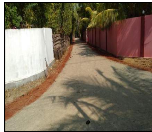
Photo of after the completion
