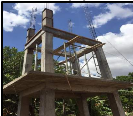
Photo of Ongoing
