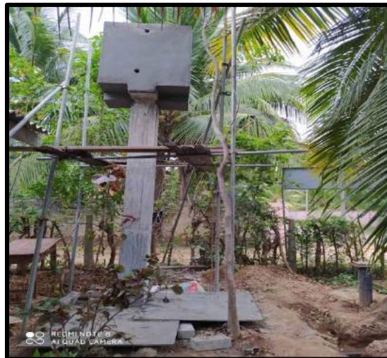
Photo of Ongoing
