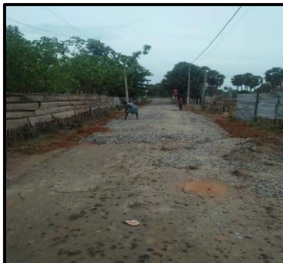
Photo of Ongoing
