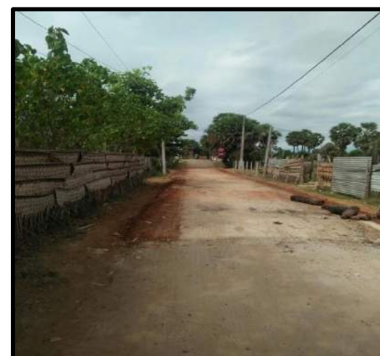
Photo of after the completion
