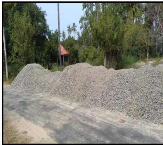
Photo of Ongoing
